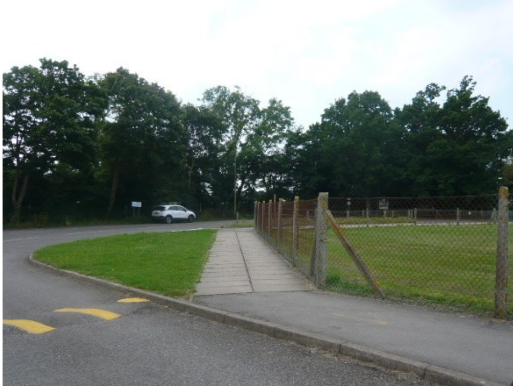
4: Existing Route of FP 62 to be diverted. New 2100mm high weldmesh fencing to be installed to replace existing Chain link fence.
