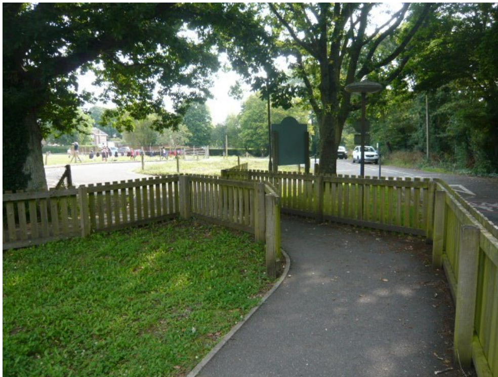
11: Existing low timber fence to be replaced with 2100mm high weldmesh fencing along outside of existing footpath, between drop off zone and end of footpath.
